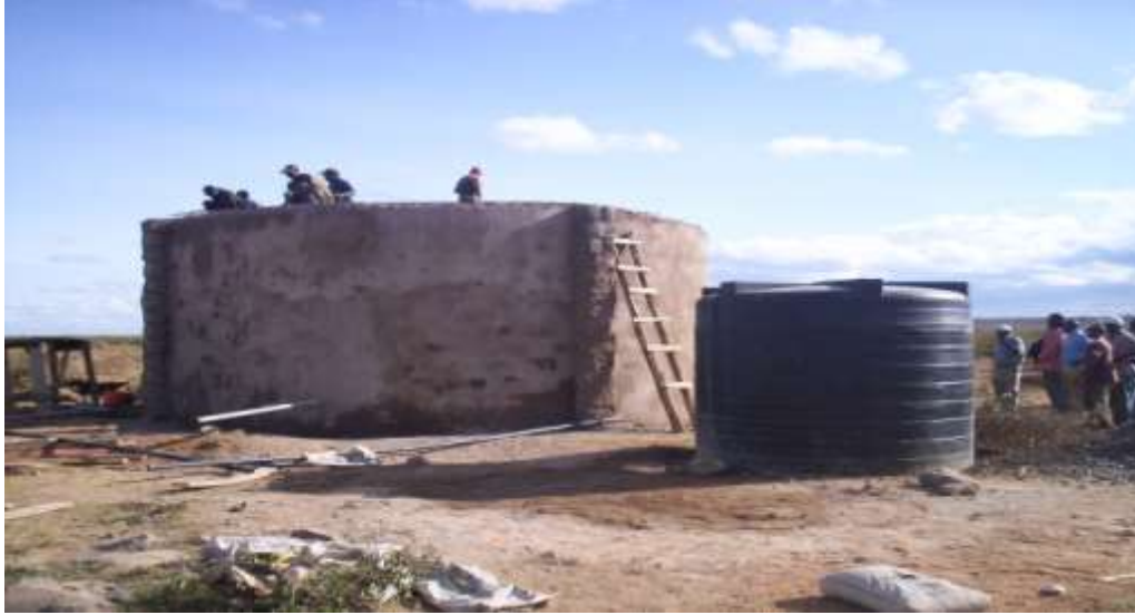
Construction of water reservoir for the pastoral nomadic community
